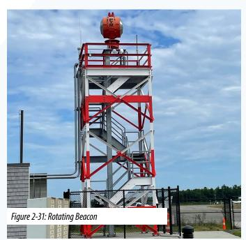
A rotating beacon, located on a metal structure adjacent to the terminal building, allows pilots to locate the airport via sequenced green and white beams of lights, which represent a civilian- land airport. Two lighted wind cones along Runway 6/24, one unlighted wind cone along runway 15/33, and an unlighted segmented circle allow users to view the wind direction, wind speed, and direction.
