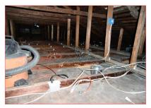
18.4 - Obsolete and suspect knob and tube wiring is present, which should be inspected and certified as safe, or replaced by a licensed electrician.
