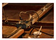
**Circuit Breakers** 5.3 - Various circuits are not labeled, which is recommended.
