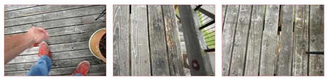
2.5 - There is no metal flashing clearance detail where the deck attaches to the house. A different flashing detail may have been used in this installation. We routinely recommend a clearance of one to two inches (visible flashing) between the deck boards and the bottom of the siding. A contractor could install a retro flashing.
