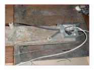
We recommend installing cover plates at all locations where they are missing.
