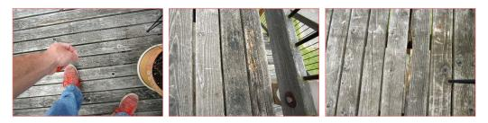
There is no metal flashing clearance detail where the deck attaches to the house. A different flashing detail may have been used in this installation. We routinely recommend a clearance of one to two inches (visible flashing) between the deck boards and the bottom of the siding. A contractor could install a retro flashing.
