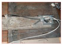
5.2 - We recommend installing cover plates at all locations where they are missing.
