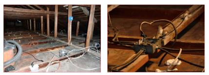
18.5 - There is unprotected electrical conduit within six feet of the attic access that is typically required to be shielded to prevent damage or a trip-hazard, and which you may wish to have serviced to comply.
