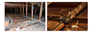
There is unprotected electrical conduit within six feet of the attic access that is typically required to be shielded to prevent damage or a trip-hazard, and which you may wish to have serviced to comply.
