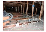
Obsolete and suspect knob and tube wiring is present, which should be inspected and certified as safe, or replaced by a licensed electrician.
